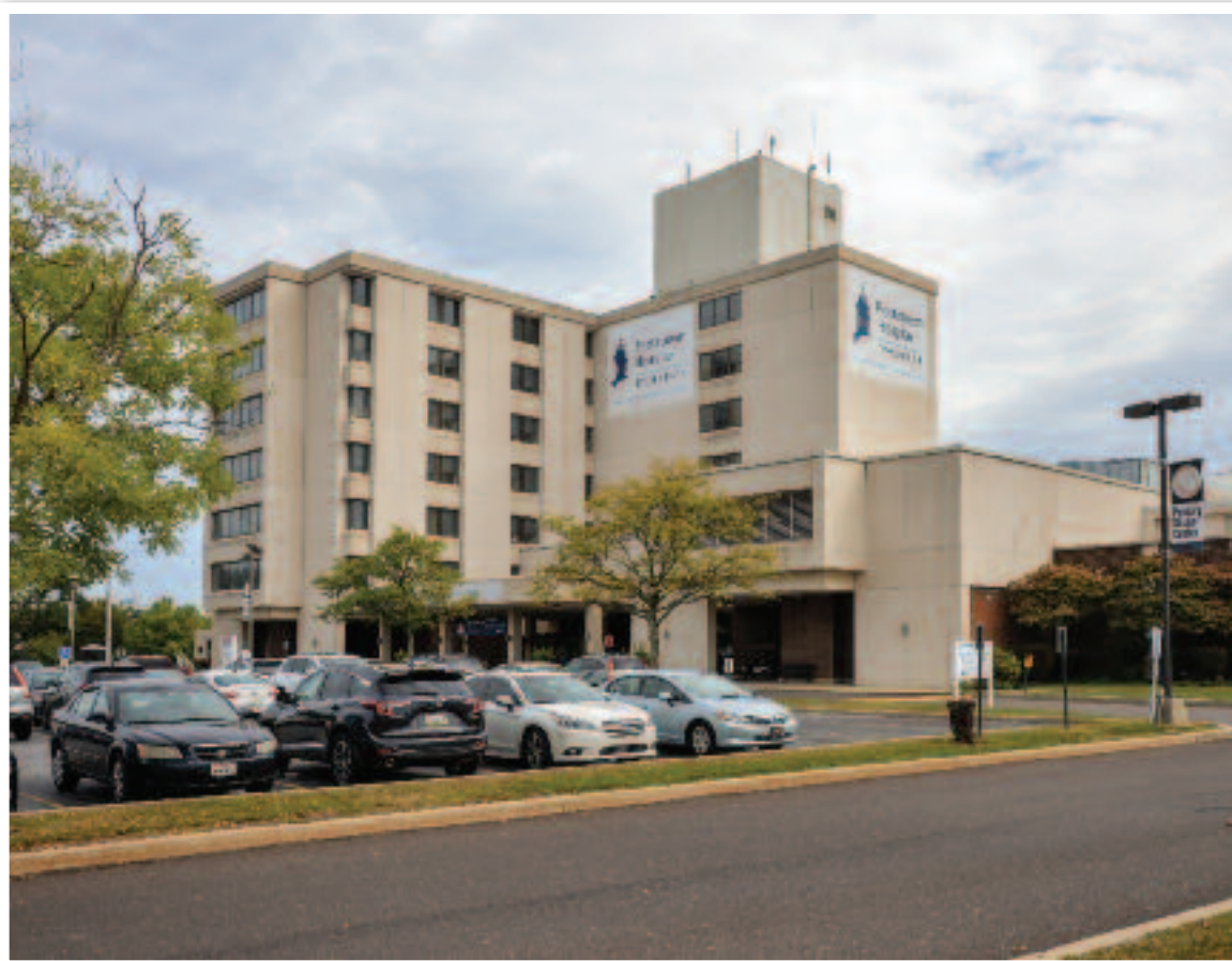
Pottstown Hospital – Tower Health located at 1600 E High St, Pottstown, PA 19464
